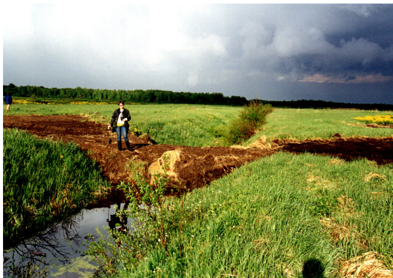
Fig. 17: Earthen dam made in the ditch (photo Taldom Administration of Specially Protected Nature Areas)
