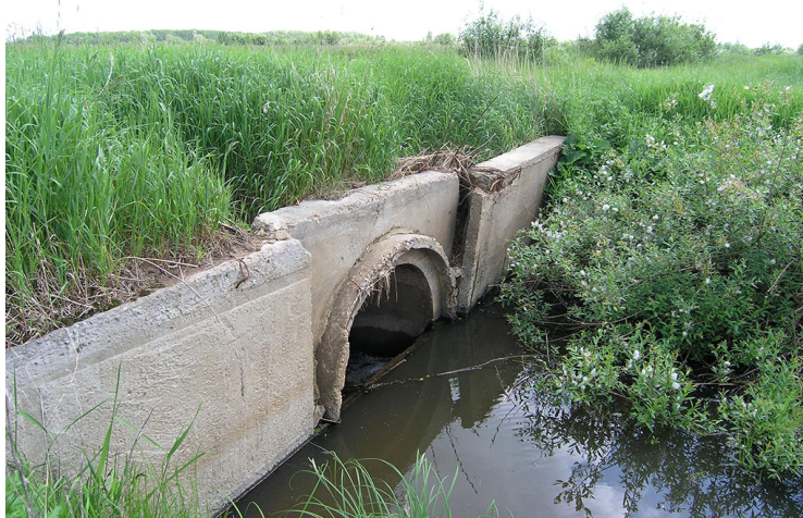
Fig. 18: Pipe in the drainage ditch with partly opened wooden gate (photo Taldom Administration of Specially Protected Nature Areas)
