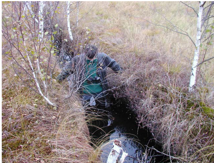
Fig. 19: One of the drainage ditches before dams were installed (photo S. Brooks)
